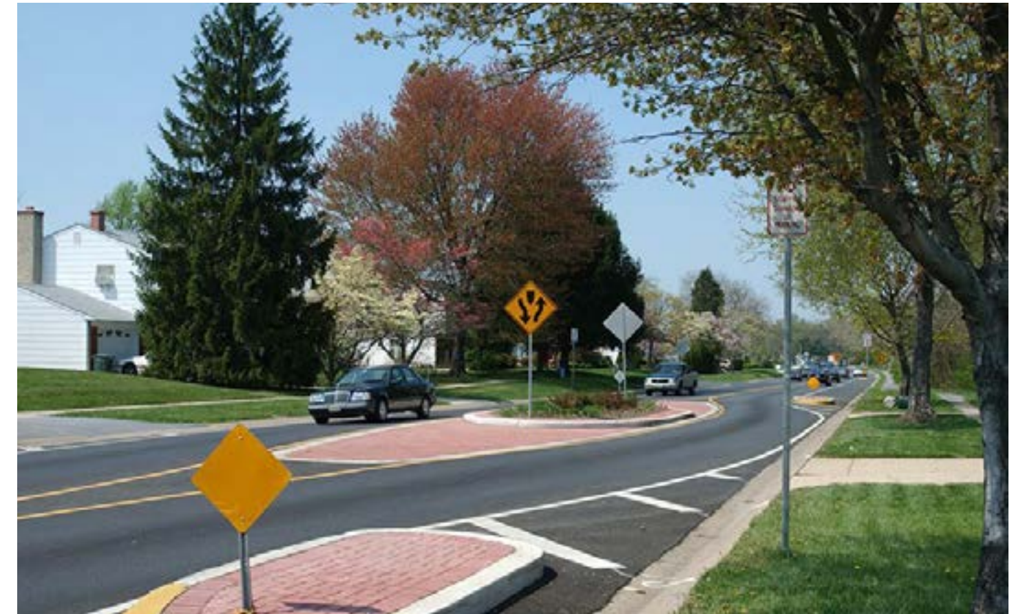
Offset curb extensions on residential or low volume downtown streets create a chicane effect that slows traffic speeds considerably. Chicanes increase the amount of public space available on a corridor and can be activated using benches, bicycle parking, and other amenities.
